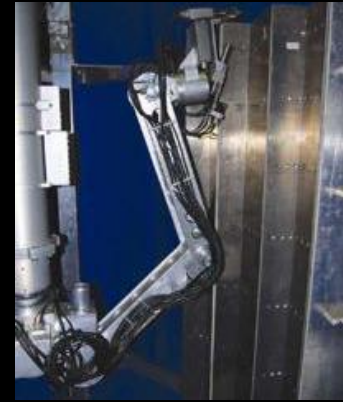
Bolt inspection robot (Westinghouse Electric Company)
