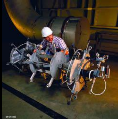
Pipe Inspection robot (Savanna River )
