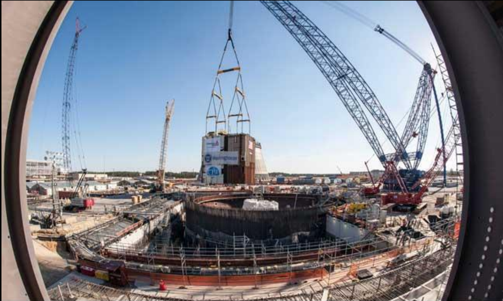
The 1,100-ton CA20 module is placed into Plant Vogtle Unit 3 nuclear island. The module, which is more than five stories tall, will house various plant components, including the used fuel storage area.
