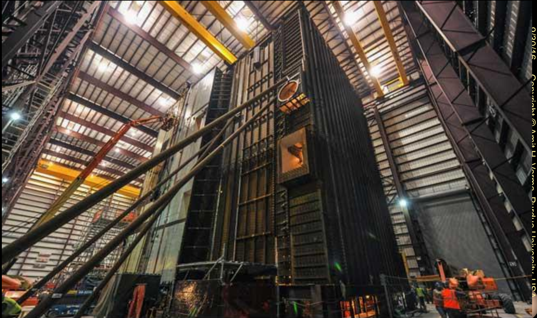
CA-20 module construction inside the Vogtle 3 and 4 module assembly building
