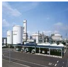
Renewable Hydrogen Production
