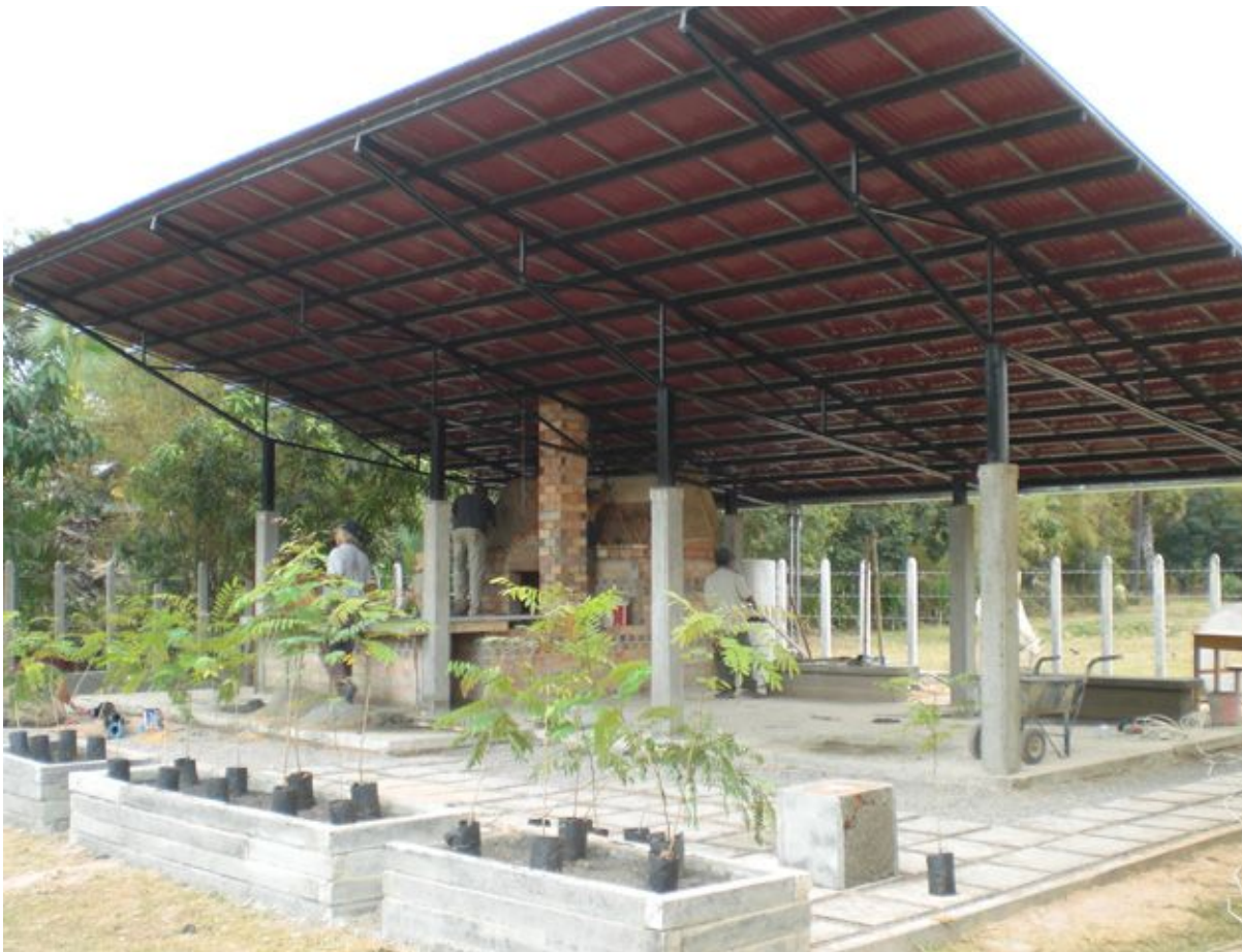
Here, team members finish building the vault that is at the core of the kitchen. A few days later, the school children were served their first meal in the new kitchen.
